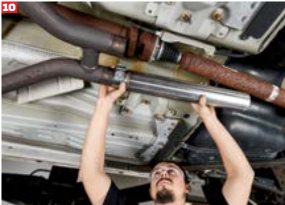
Using the supplied clamps, Weathers loosely installed the Hooker BlackHeart connector pipes over the OEM H-pipe.
